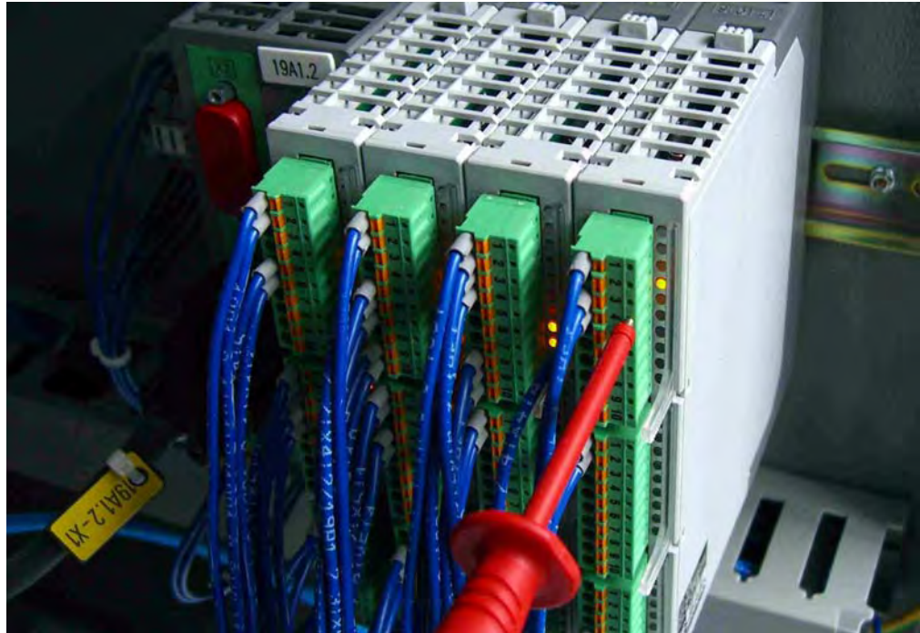
Figure: Measuring at a terminal of the I/O module PLD 16-8 using a needle tip probe
