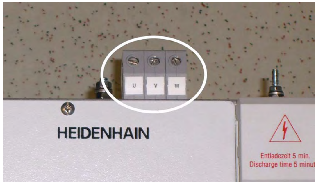
Figure: Primary connection on the UE 241 B compact inverter
