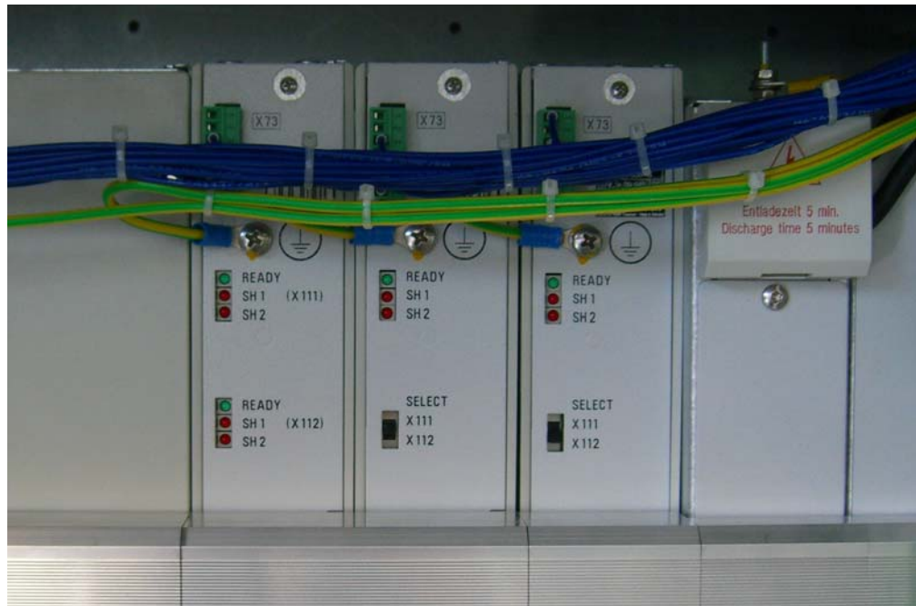
Photo: LEDs on the HEIDENHAIN expansion boards
