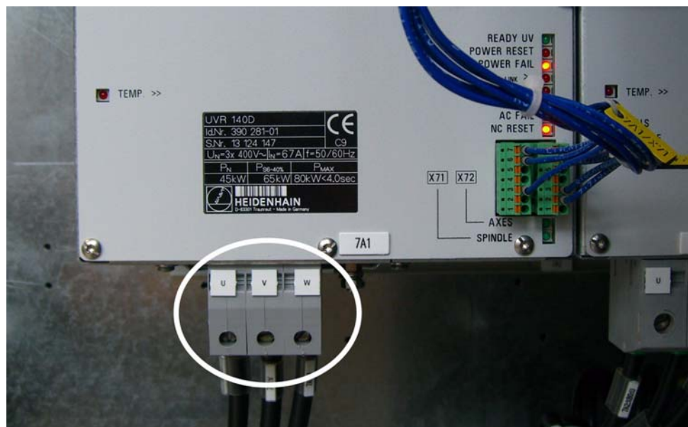
Photo: Primary voltage connector on the UVR 140 D power supply unit
