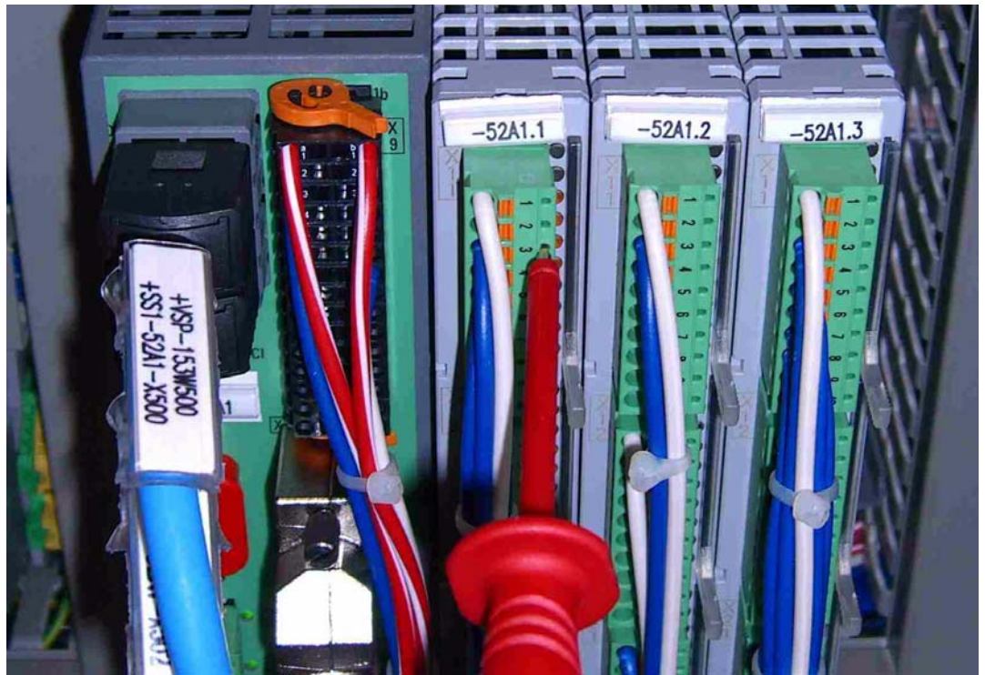
Figure: Measurement at a terminal of the I/O module PLD-H 16-08-00 using a needle tip probe
